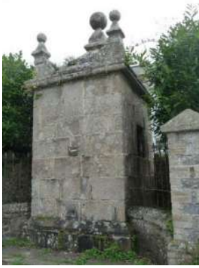
Water Supply Conduit, Brownston Street, 1708.
